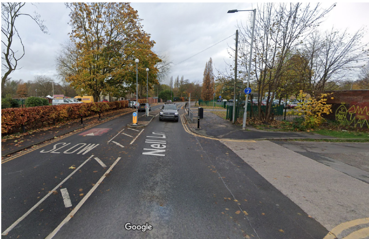
Continuing double yellow lines, slow markings, cushion painting, footway bollards and lit crossing point.
